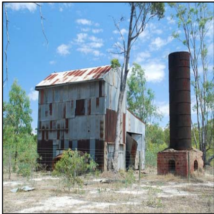
(a) Remnants of corrugated iron battery shed & iron chimneystack, at Bombay mine
