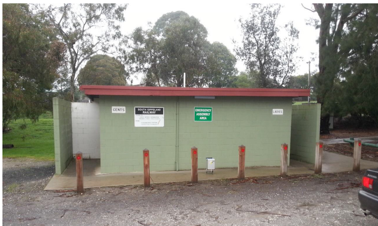
Photograph of Control Station 201406500001
