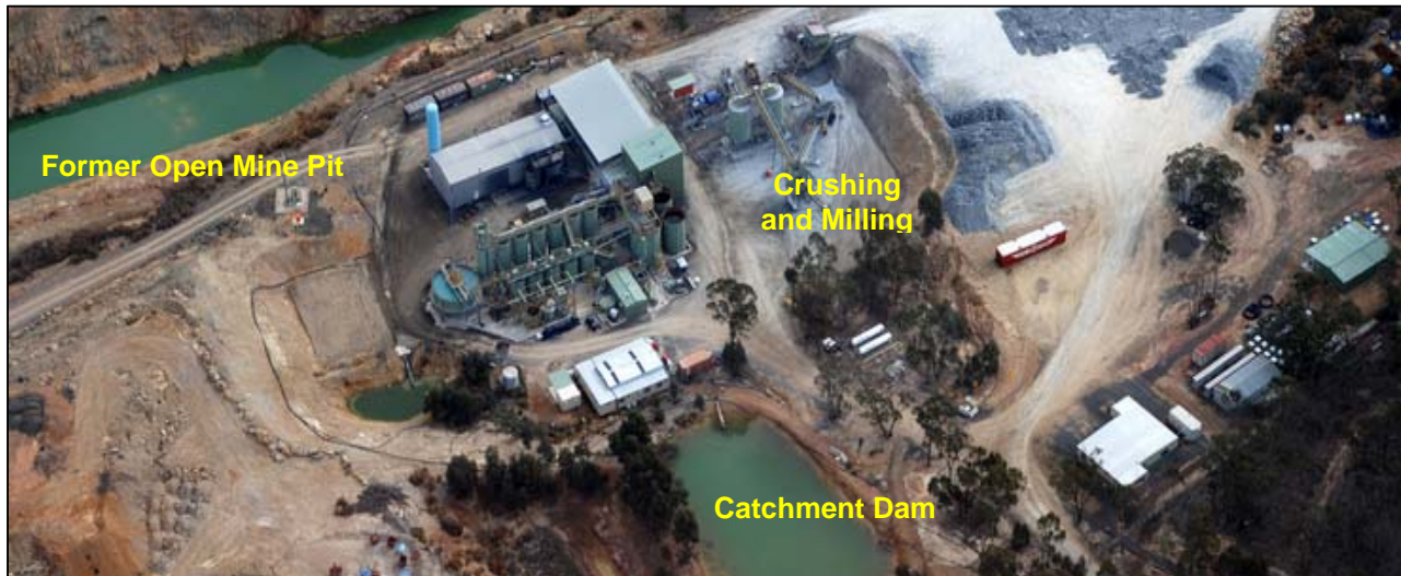
Figure 18: The Brunswick Processing Plant (Mandalay Resources, 2012)
