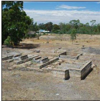
(b) Remnant footings at Costerfield Main Shaft
