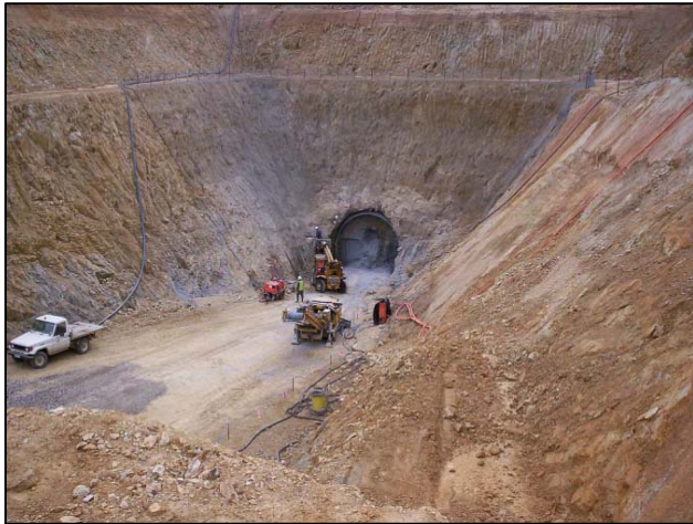
(a) Augusta Underground Mine
