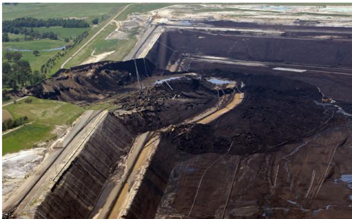
Figure 3.3 : Yallourn Mine batter failure (Photo source: theage.com.au online)
