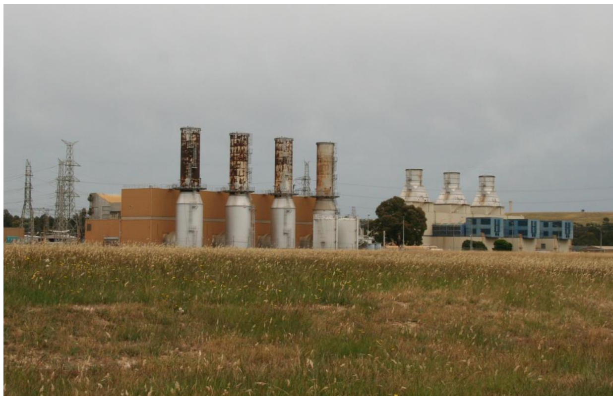
Figure 5.5 : Jeeralang gas fired power station (Source: By Marcus Wong - Own work, CC BY-SA 3.0, https://commons.wikimedia.org/w/index.php?curid=5567823 )
