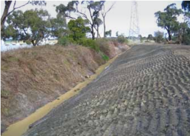
Reclaimed quarry face, cross ripped and hydroseeded.
